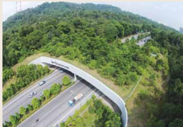
The Eco-Link@BKE in 2015, a bridge constructed in 2013 for wildlife to cross from the Bukit Timah Nature Reserve to the Central Catchment Nature Reserve
