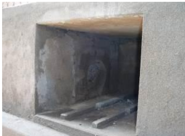
Figure 3.14: Pangolin den without bedbox; circular entrance for pipe at the side of the den, ribbing on the floor to prevent the bedbox getting wet if flooding occurred.
